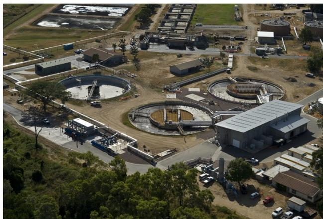
The process consists of two MBR streams that have been constructed through the modification of existing secondary clarifiers.
