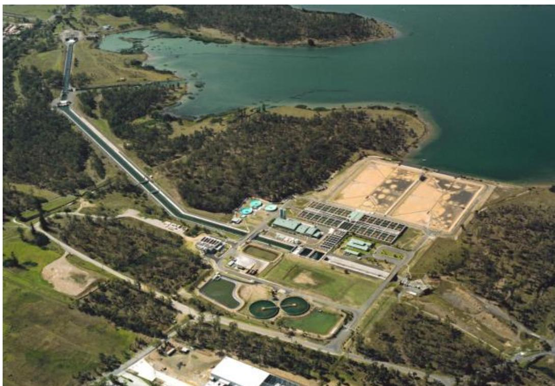
The plant uses chemicals in the water treatment process, involving the addition of flocculants and pH adjustment chemicals prior to filtration. The filtered water is fluoridated and disinfected with chlorine and ammonia. The chemicals used for the treatment process are transported to the site in road tankers and unloaded into bulk storage containers located on the site.
