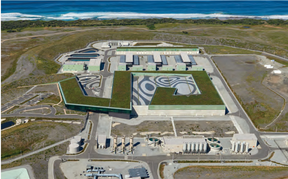
The Victorian Desalination Project is home to one of the world's largest reverse osmosis desalination plants.
